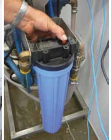
Hand tightened back on, then push in the bleeder valve to release excess air, hold until you get water.
