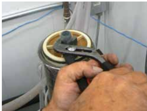
After the collar is off, grab the nipple on the filter with your plumber's pliers and turn and pull at the same time.
