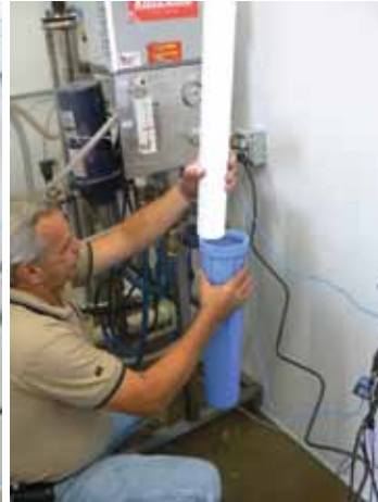
Take out the old filter and swap with a new one.
