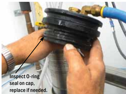
Before placing the cap back on, check the O-ring seal on the cap and replace if needed.
