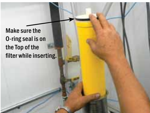
Insert your new filter into the membrane. Be sure the O-ring seal is at the TOP when inserted.
